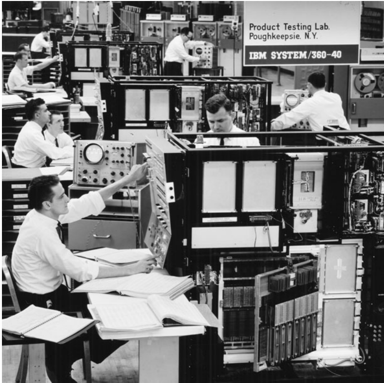
FIGURE 1.10 Engineers test processors for the System/360 Model 40, a medium-sized IBM mainframe introduced in 1964. (Courtesy of International Business Machines Corporation)
