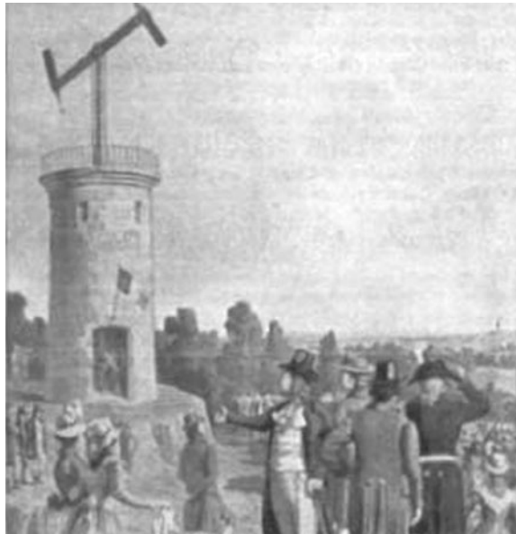
FIGURE 1.12 A semaphore telegraph tower on the first line from Paris to Lille (1794). (Photo l'Adresse Musée de La Poste, Paris / La Poste)
